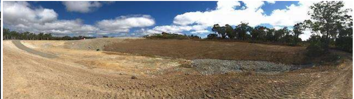
Significant Environmental Improvement Works were undertaken at Marulan Landfill in 2017/18.
