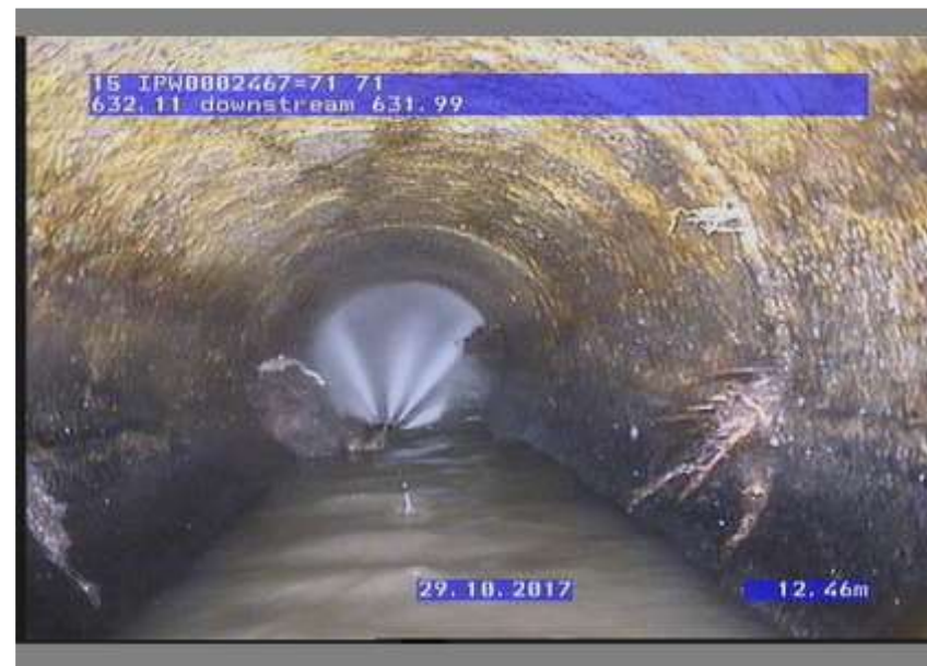
Figure 1 - Sewer relining equipment
